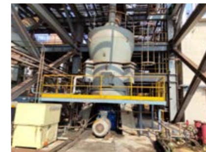
Commissioning of PCI (18 TPH) & O2 Plant (3000 Nm3)
